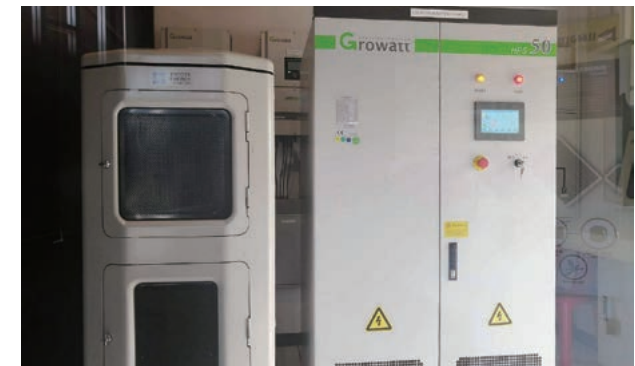
A power storage system that reuses End-of-life HEV batteries
